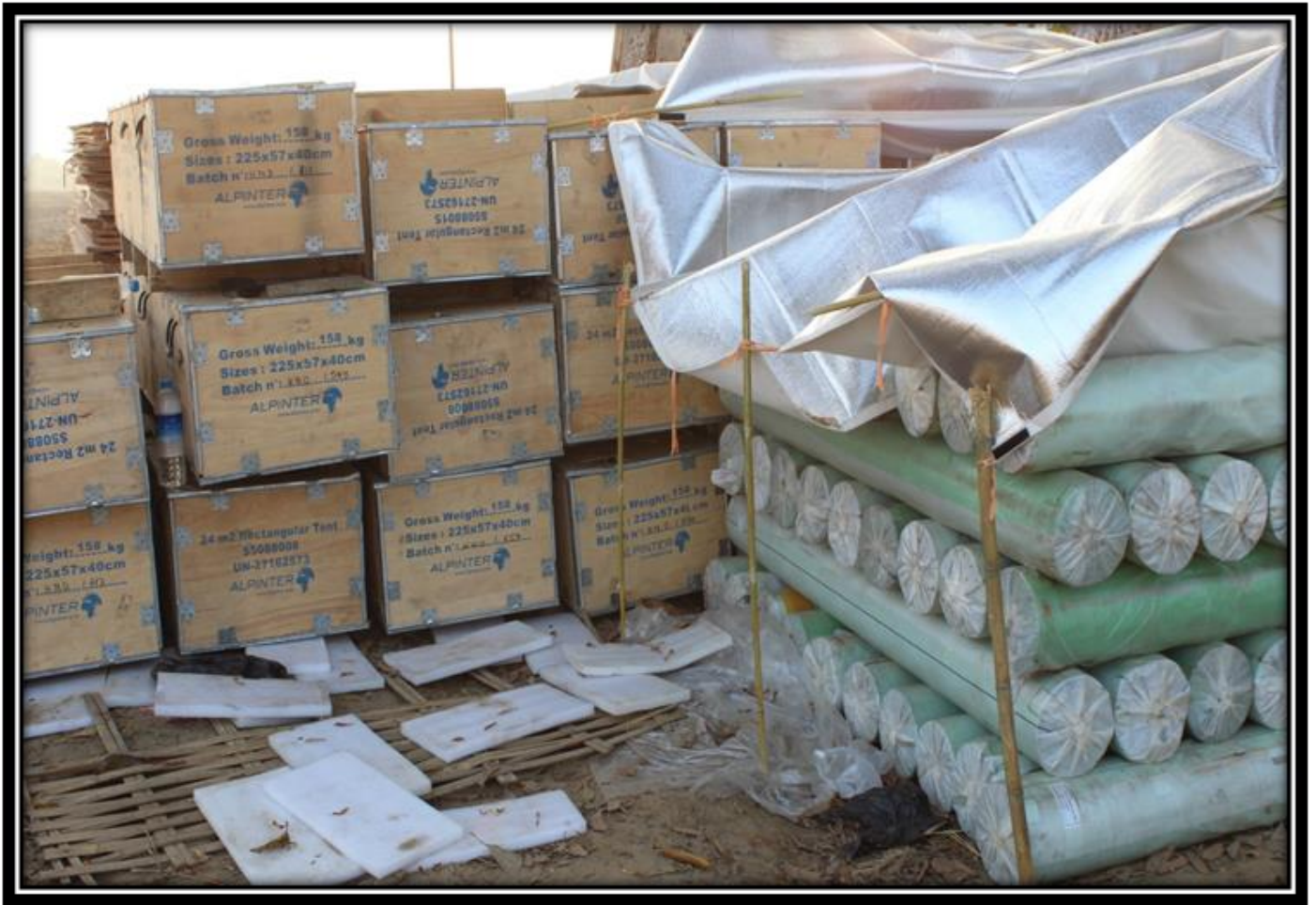
Heaps of the accessories for construction of temporal shelters at Hla Poe Kaung Village
