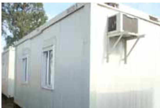
Containers for staff accommodation at the Bunia field office, DRC © ICC-CPI
